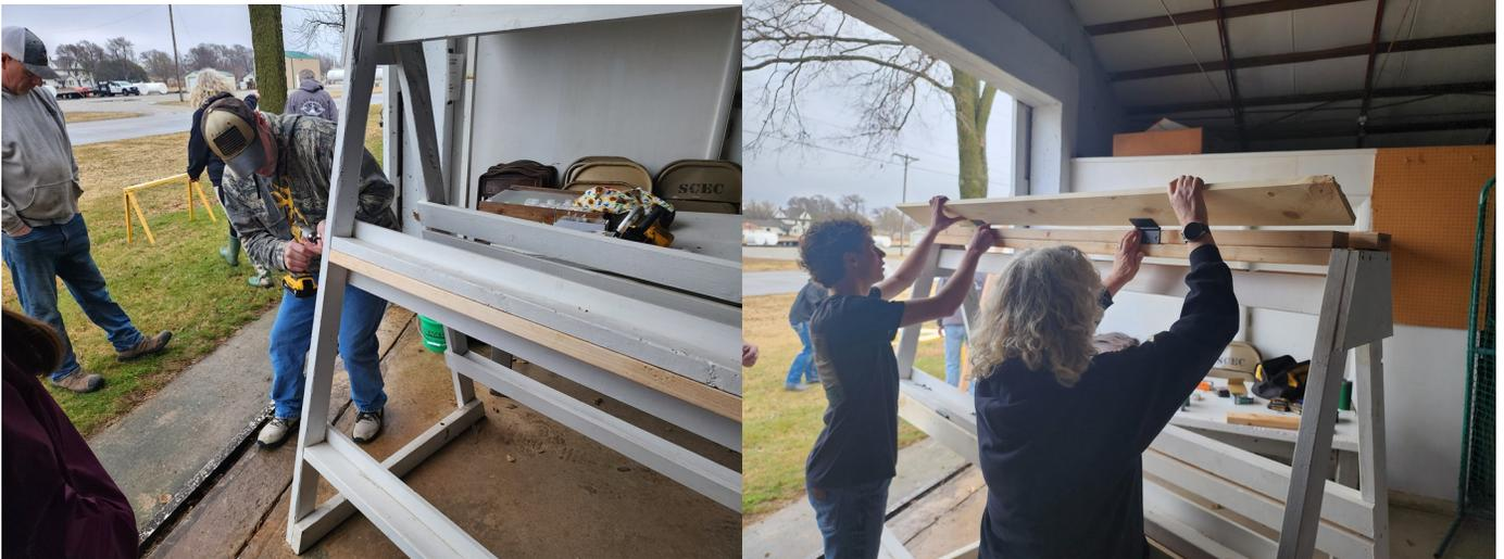
On these shelves in particular, a 2”x4” was added to the top of each shelf to prevent the Plexiglas from being slid upward while boxes rested on the rack. Then 1”x3” and 1”x6” boards were added with hinges to each shelf to prevent boxes from being taken off the rack. A combination lock will be installed at the end of the shelves on the wood flaps and a more simple locking mechanism on the other end. Each county may have a unique set of shelves that can be modified with a little ingenuity.
